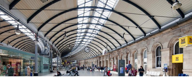
All of the original building structure from 1850 was retained. The contemporary construction was placed inside, with care given to ensure minimal contact with the existing structure.
